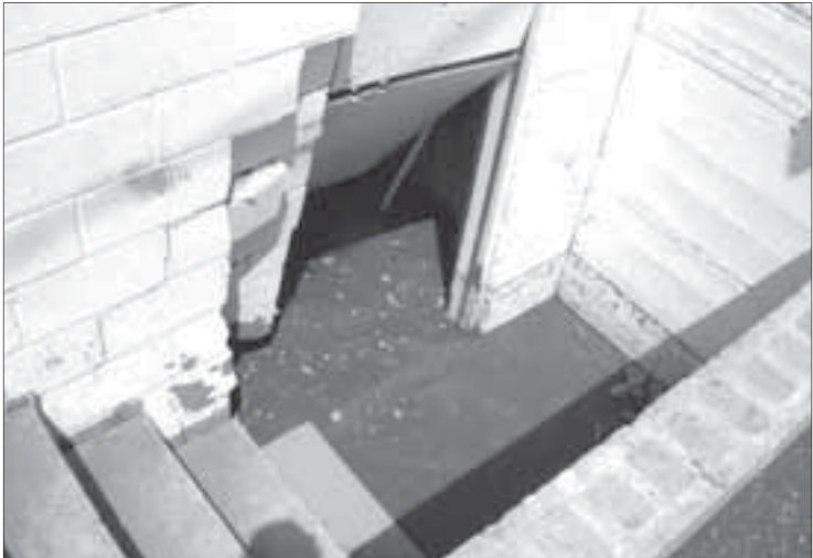
Rushing water from the last week’s flooding collapsed a rear wall on the American Legion Post 32 Hall in Homedale. Submitted photo
